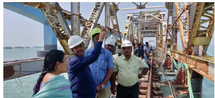
Fig. 4: Prof. Kapuria inspecting the preparation for testing of Pamban Railway bridge with moving train for its structural integrity assessment.
